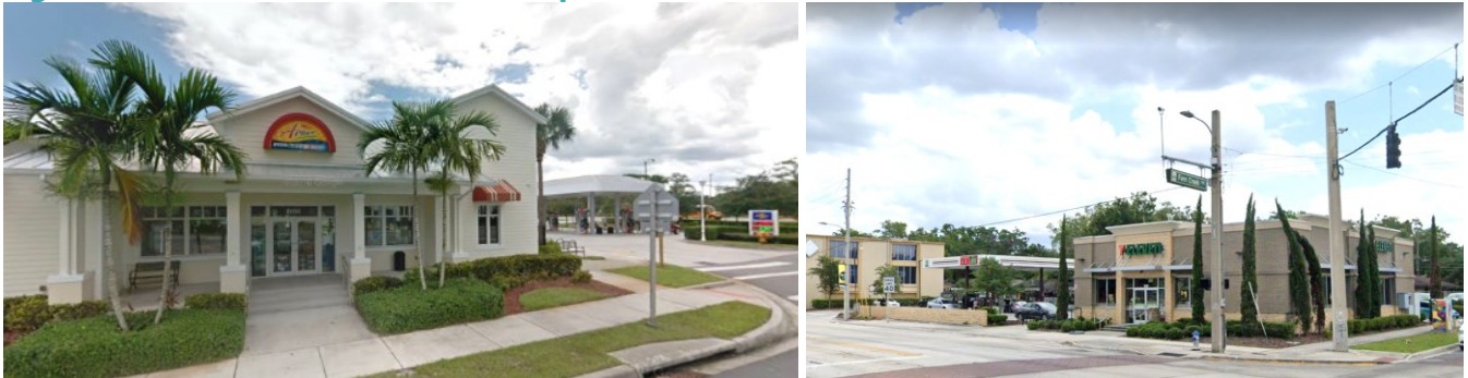
Gas Station main facade with pumps to the side of the building
