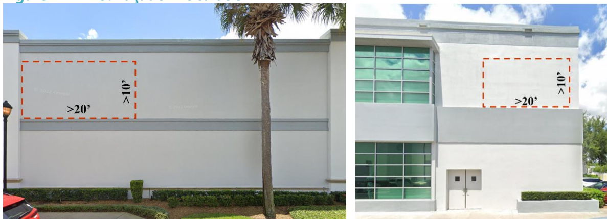
Examples of blank wall exceeding 20 horizontal feet by 10 vertical feet without articulation
