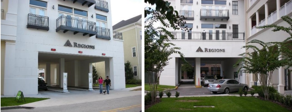
Figure XIV - 46. Interior Drive-Through Facilities
