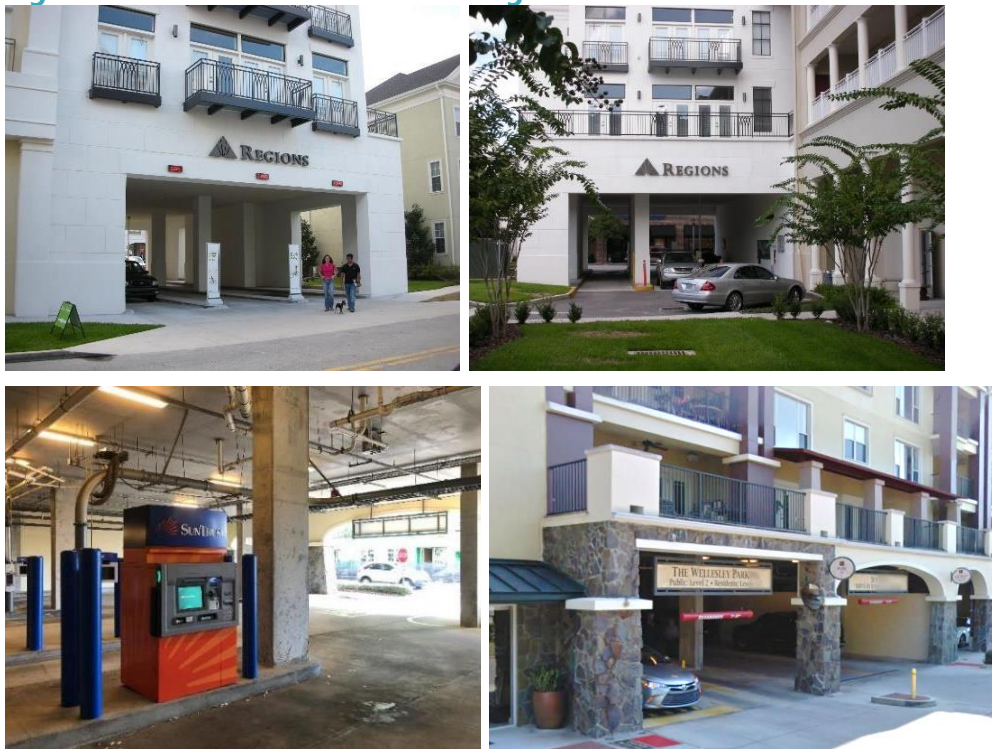
Figure XIV - 47. Interior Drive-Through Facilities
